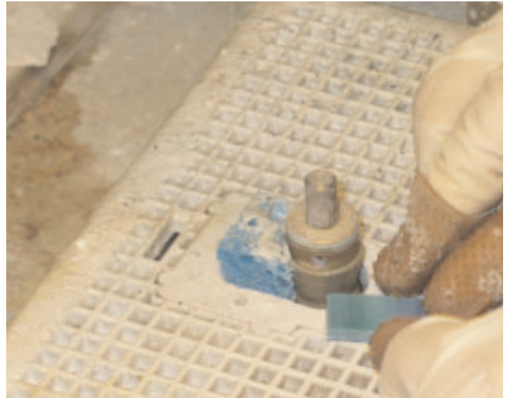
3. All the edges are ground and shaped to fit.
